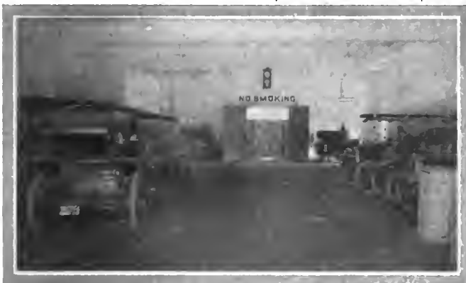
GROUND FLOOR OF GARAGE SHOWING ENTRANCE TO ELEVATOR.
